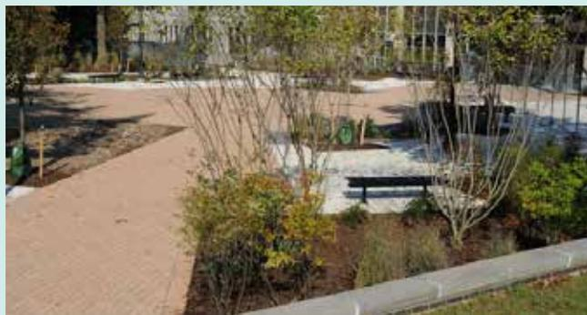
**Porous Paving** can be configured to either allow water to infiltrate through the paver joints or through the paving itself. As with the other systems described above, porous paving is installed over a base of broken stone.
