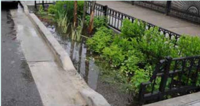
**Right of Way Bioswales and Stormwater Greenstreets** are planted areas in a sidewalk or roadbed that capture curb runoff. They are installed over a layer of broken stone with engineered soil and topped with appropriate plants and trees.
