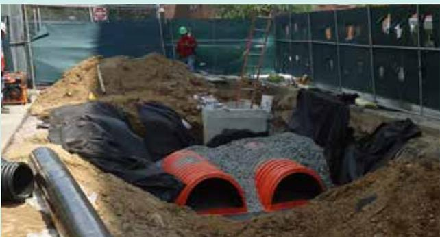
**Subsurface Infiltration Systems** are installed underneath parking lots or other large paved surfaces. They include a bed of broken stone and a storage system, such as storm chambers or perforated pipes.
